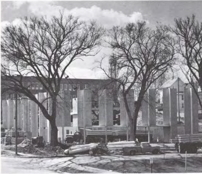
Construction is well under way on the new pre-cast building for the Greeks.
